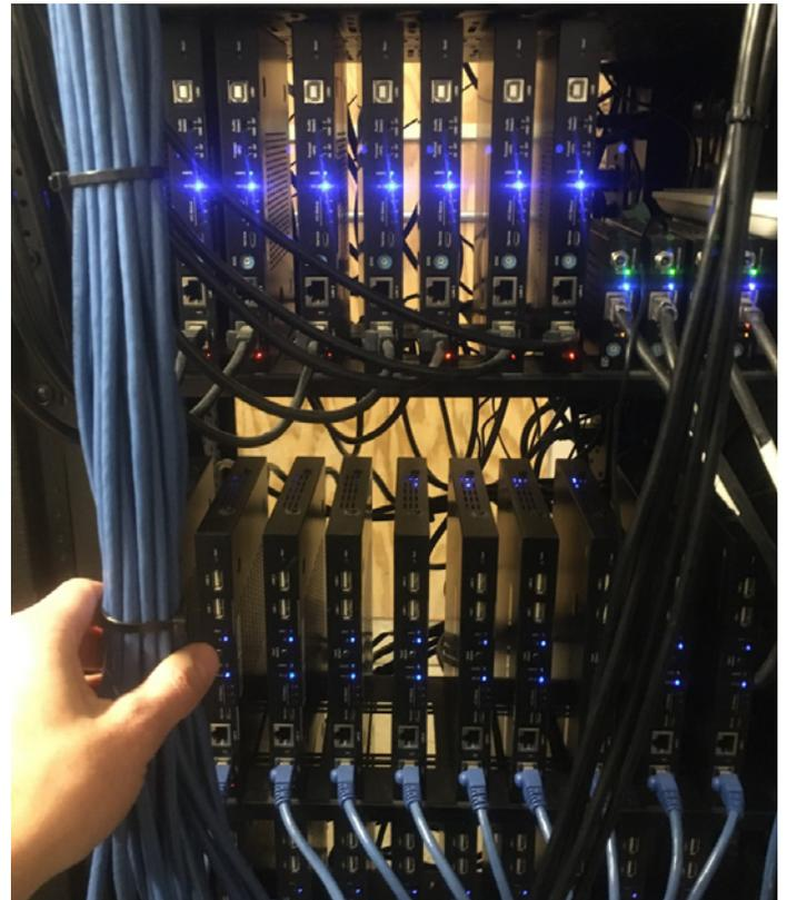
Central to the restaurant's needs but unconventionally not centrally located at the projectors, the unique layout and design feel of the dining room required the AV over IP decoders to bypass traditional placement at the displays and instead be housed at the equipment rack located one floor above. Thanks to Key Digital's [KD-X444L long range extenders](#), the installation had room to travel up to 100 meters in distance while upholding pristine video quality.
